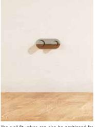
The wall-fit valves can also be positioned far from the radiator; the important thing is that they are installed lower than the water inlet of the radiator.
